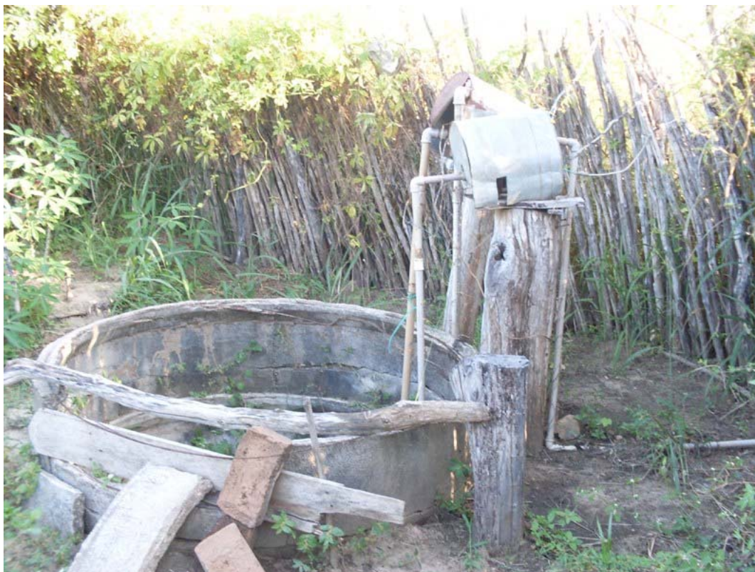
Figure 4.51: Amazon-type well that provides water to the community of Reconquista.
