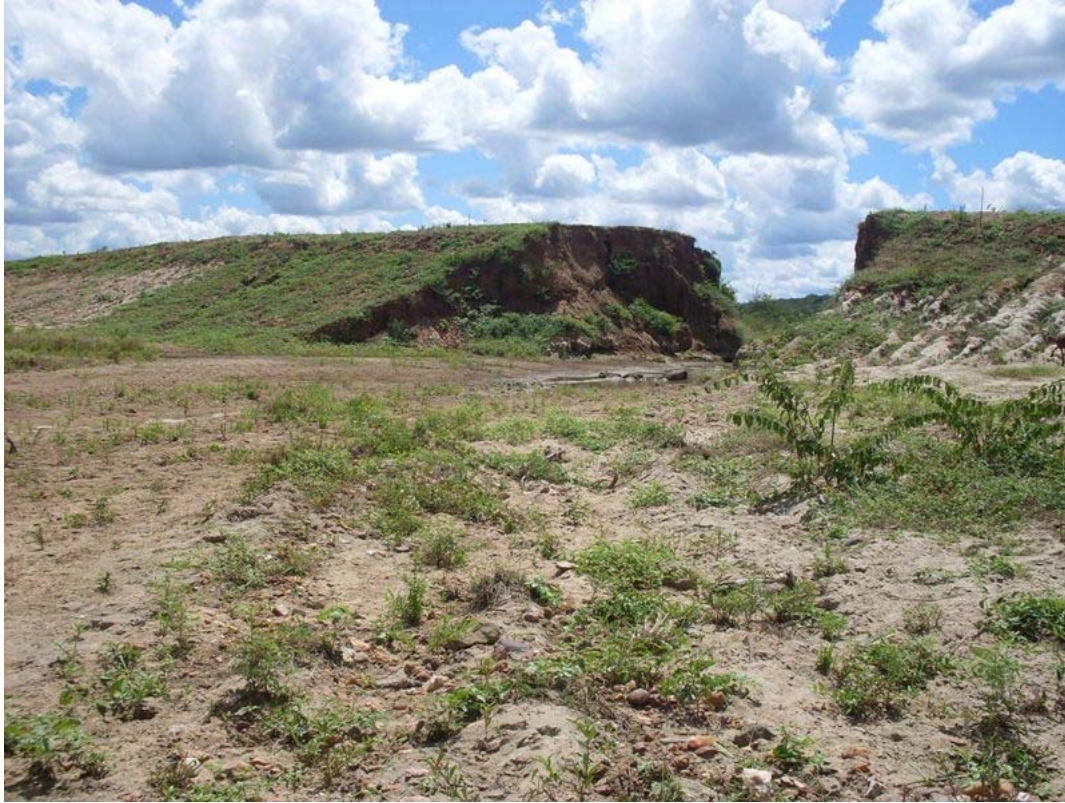
Figure 4.121: The Tanques reservoir, which cracked during the March 2009 flood.
