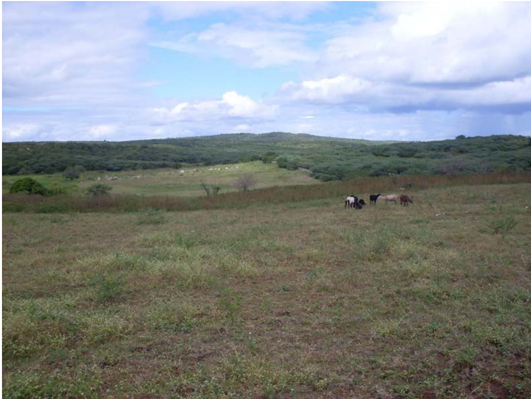
Figure 4.32: A general view of the abutment, left to right, of the mouth of the Lagoa Nova Dam.
