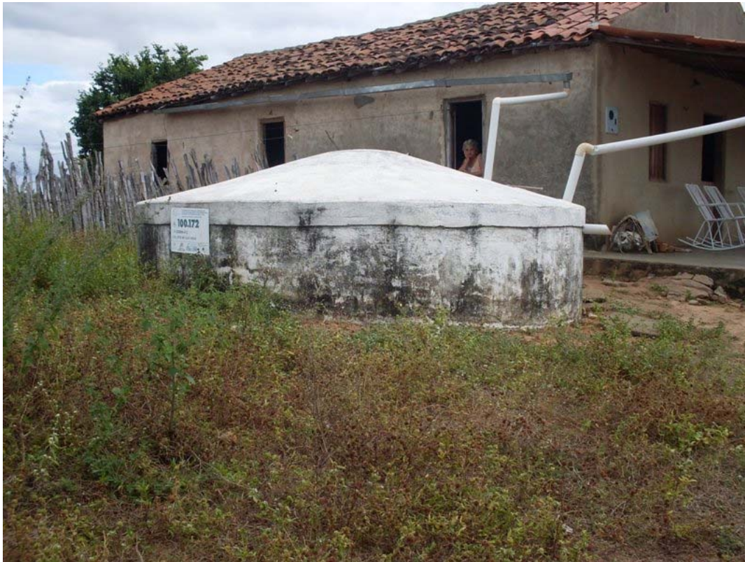
Fig. 4.162: Rainwater cistern in Amanaju 01.
