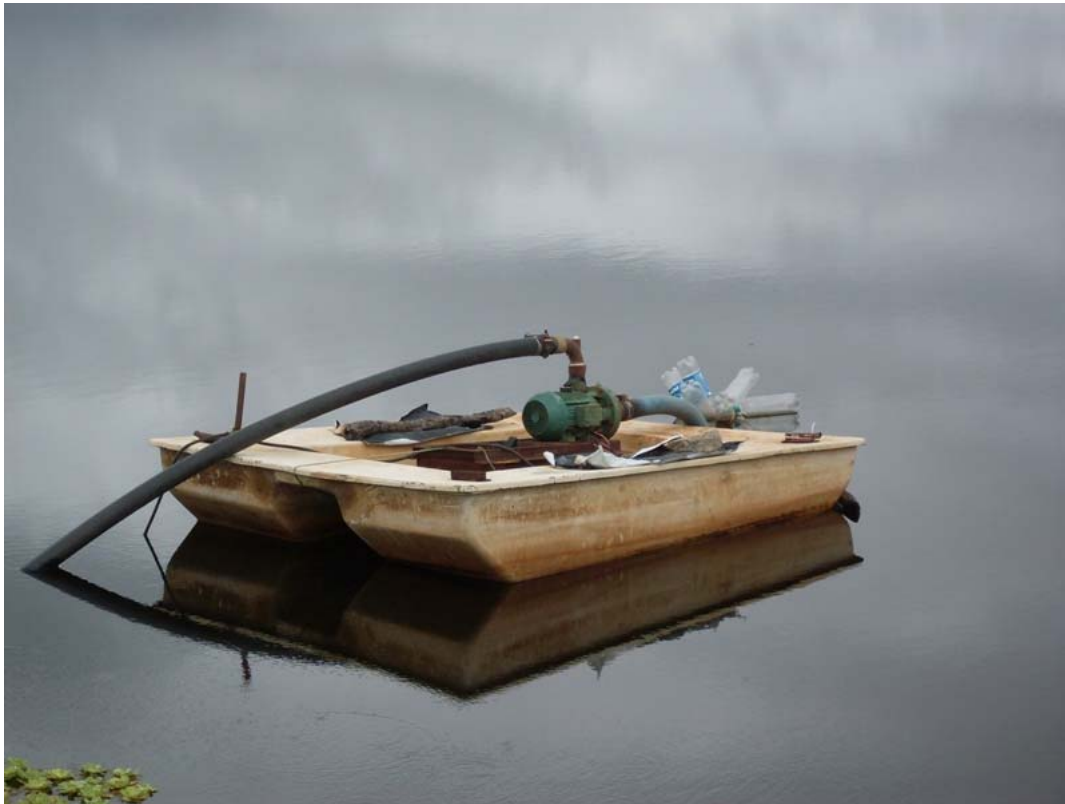
Figure 3.9: Floating water collection for Carnaubinha at the Quandu reservoir.
