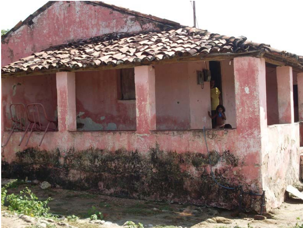
Figure 4.7: House in the community of Alto Santo supplied by the Açude Novo aqueduct. The meter can be seen outside the house.
