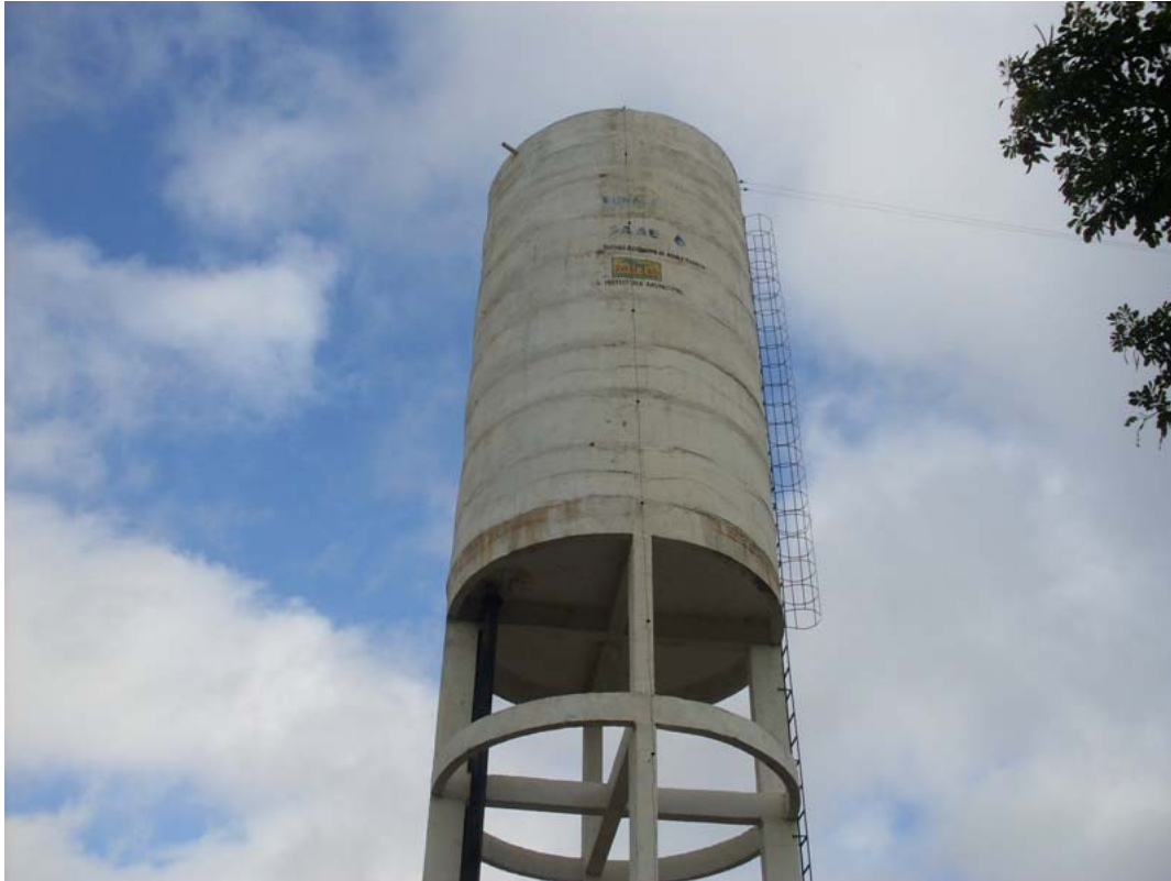
Figure 4.140: 200 m 3 elevated reservoir in Milhã's town center.
