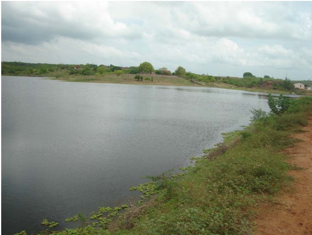
Figure 3.7: Riacho do Meio Reservoir, with the ETA in the back, to the right.
