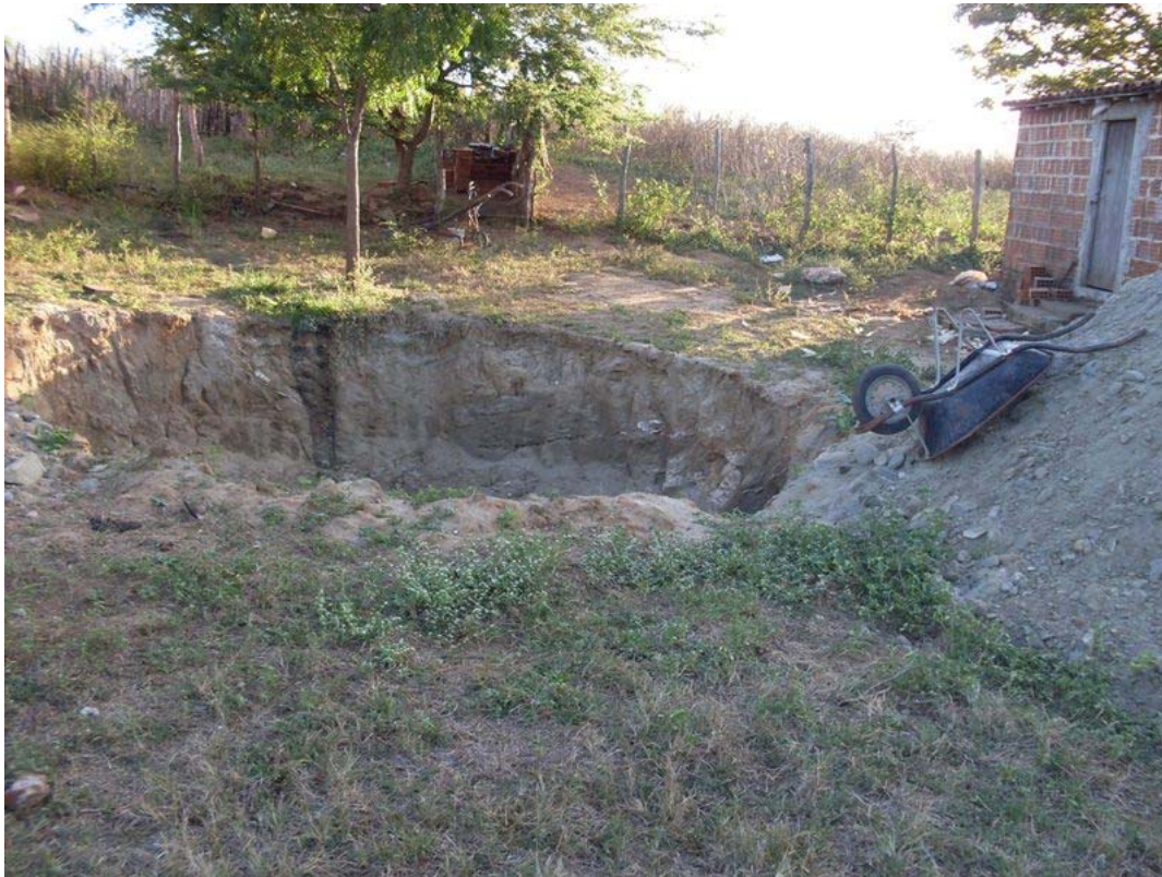
Figure 4.102: P1MC Cistern under construction in the community of Macaco.
