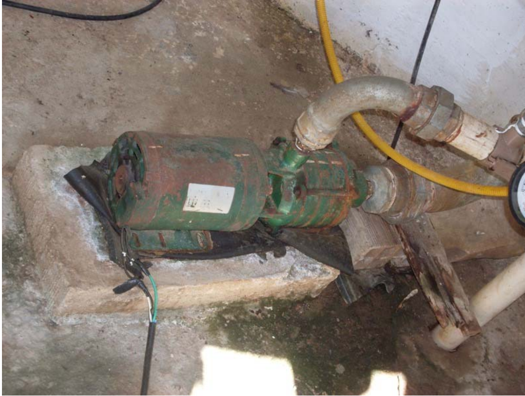
Figure 4.11: Pump used to deliver water from Açude Novo to the communities of Grosso, Tabuleiro and Furnas.
