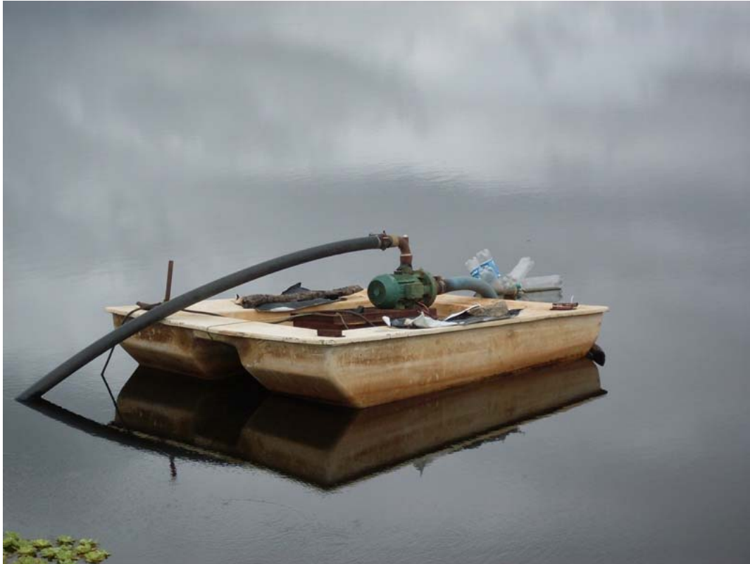
Figure 4.2: Floating water collection device in the Quandu reservoir to provide water to Caraubinha - 5 HP.
