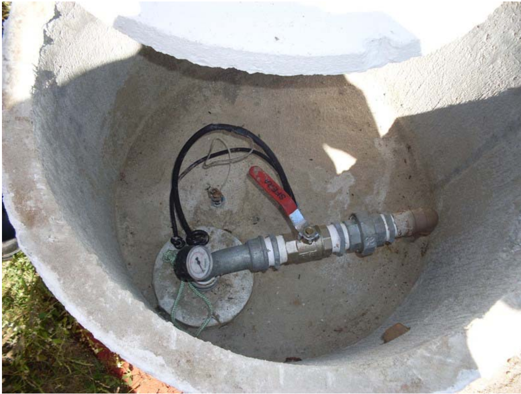
Fig. 4.160: Deep well in Barra 01.
