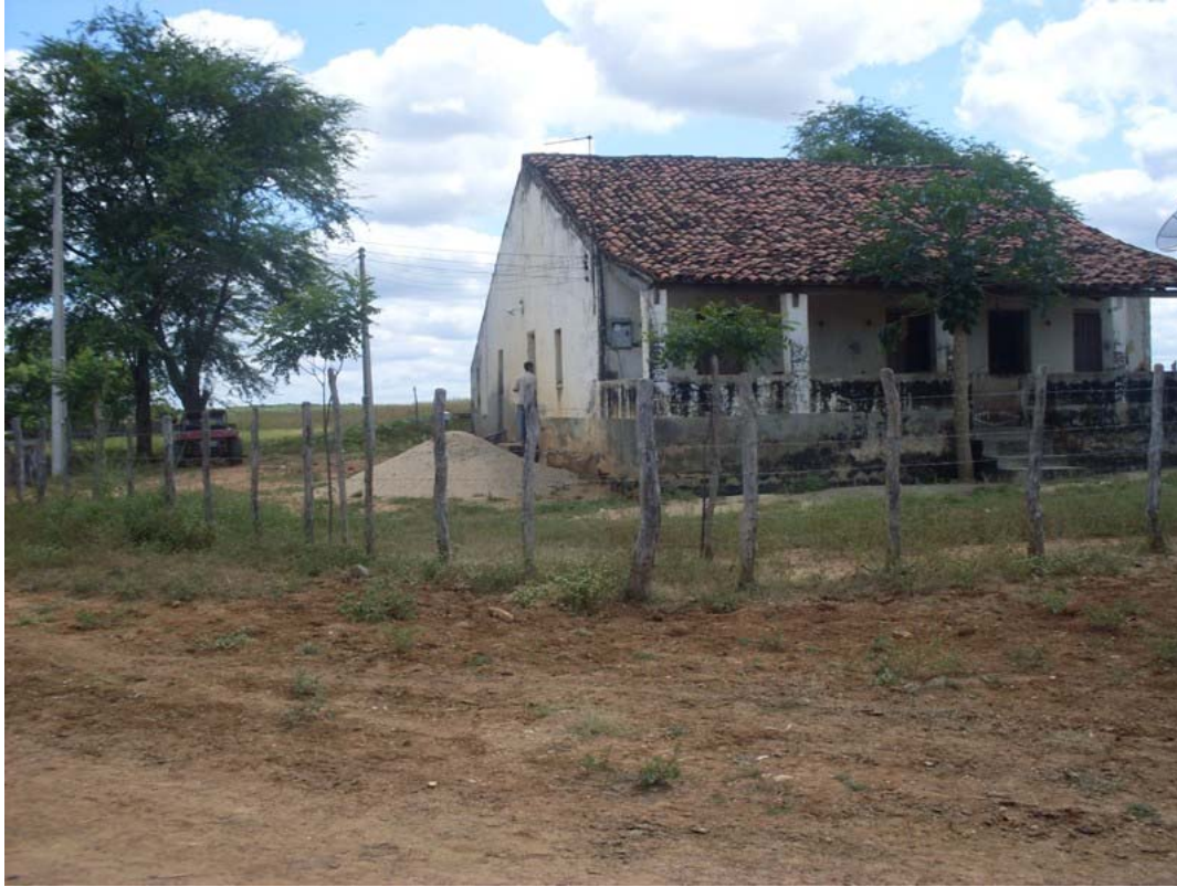
Figure 4.82: Homes in the community of Sabonete.
