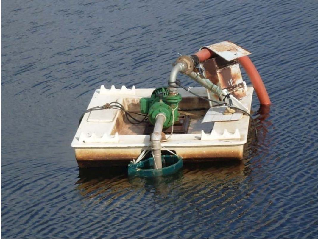
Figure 4.134: Floating water catchment to provide water to Milhã.
