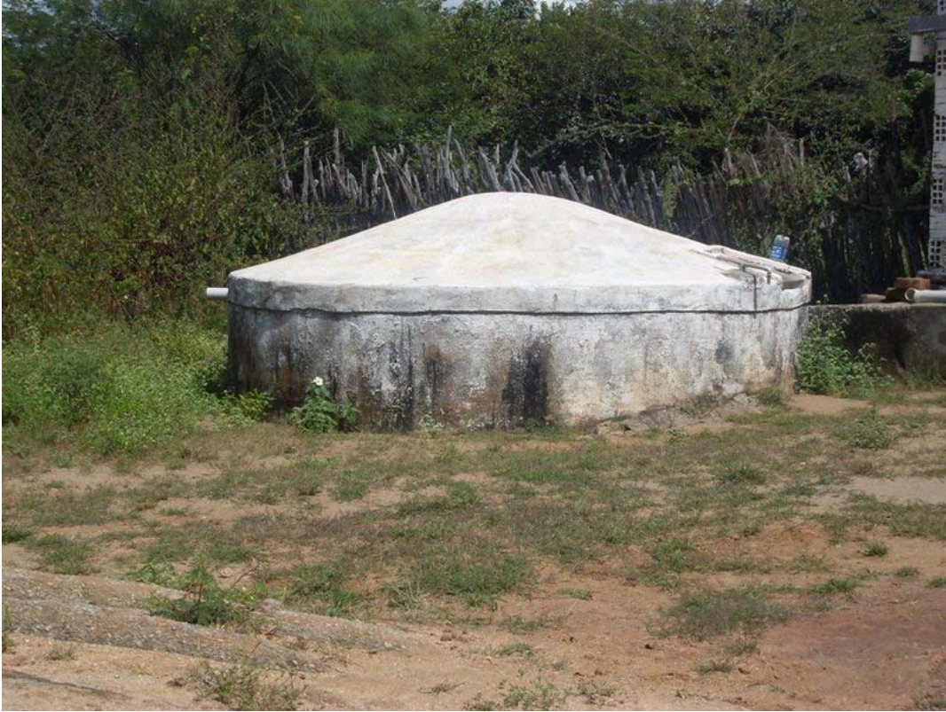
Figure 4.80: Rainwater cistern as an alternative source of potable water in Esperança.
