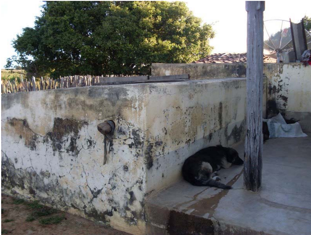
Fig.4. 152: Masonry cistern built by Milhã's Municipal Government in Morada Nova.
