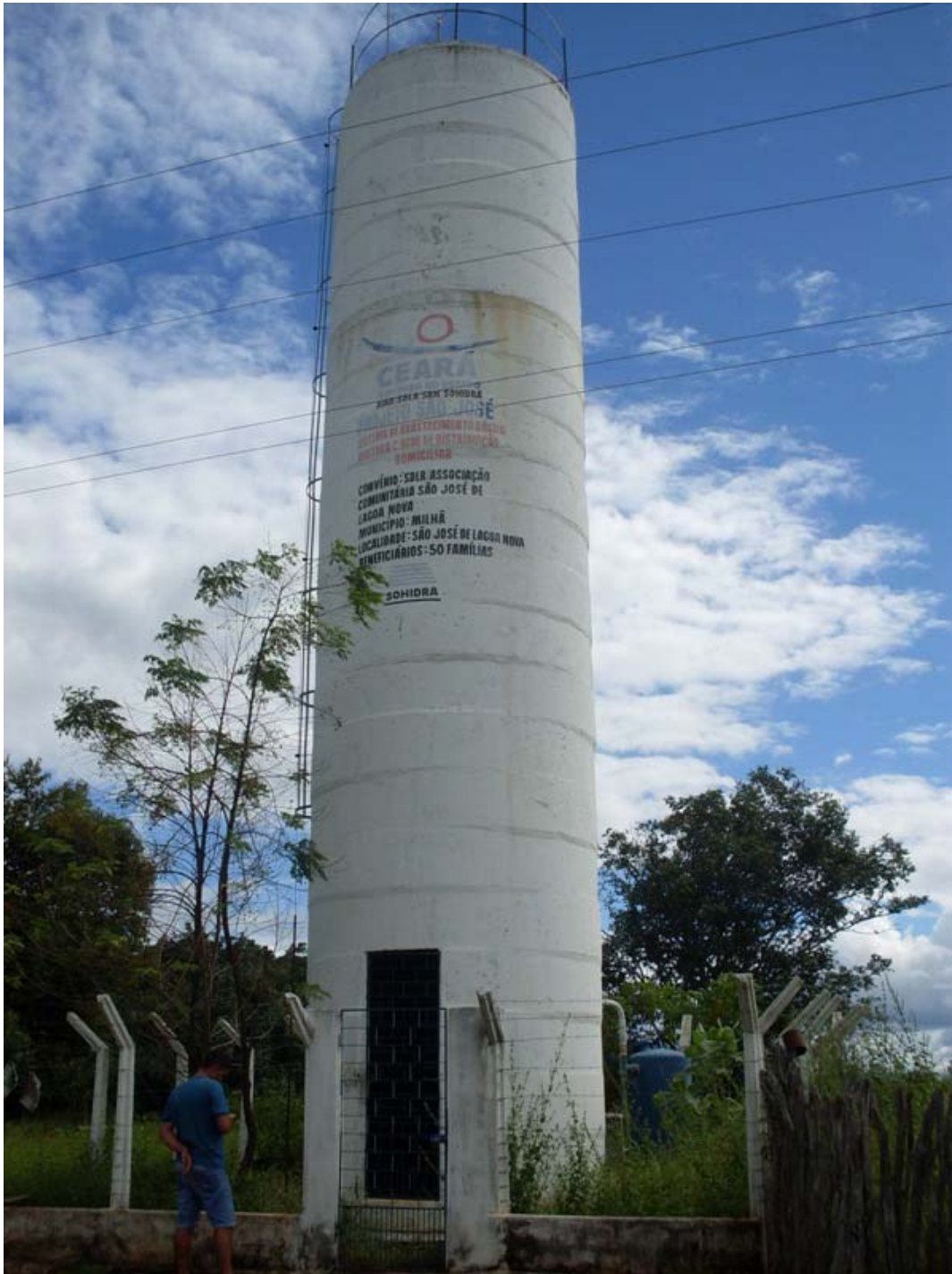
Figure 4.29: Lagoa Nova's Elevated reservoir.
