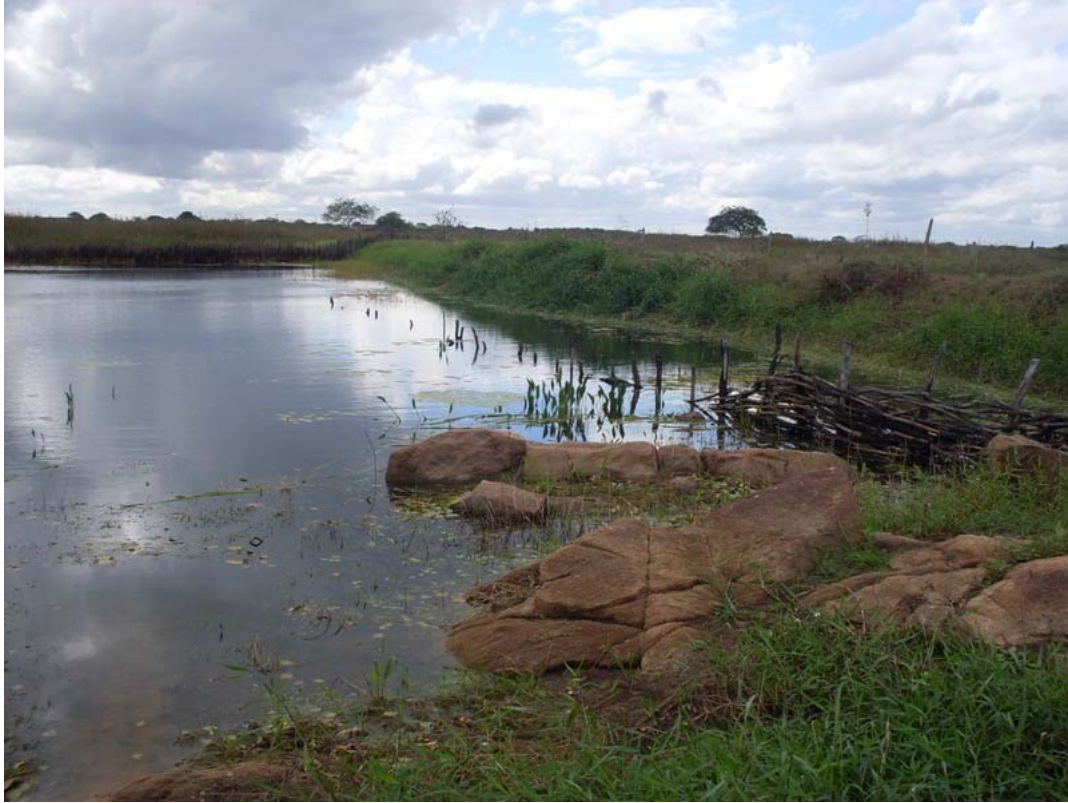
Fig.4. 159: Mr. Almino Alves' reservoir in Barra 01.
