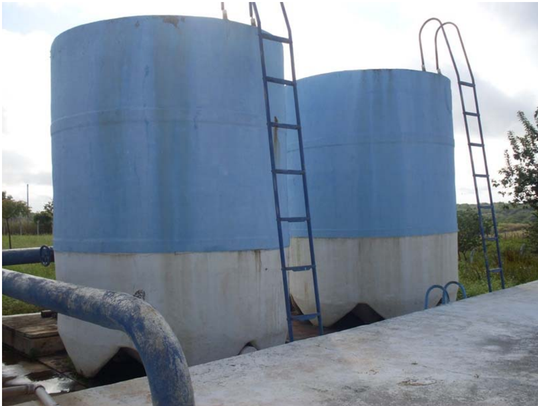
Figure 4.137: Filters at Milhã's ETA.
