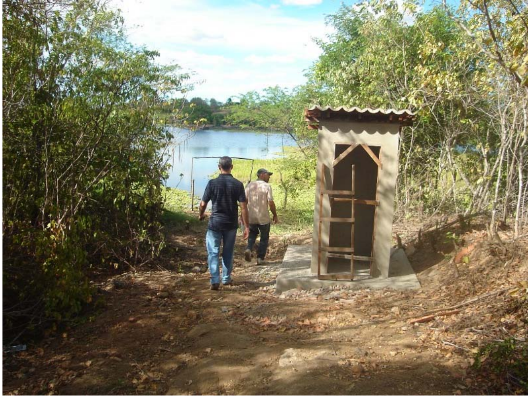
Figure 5.22: Pump house at the collection site at Riacho do Meio reservoir.
