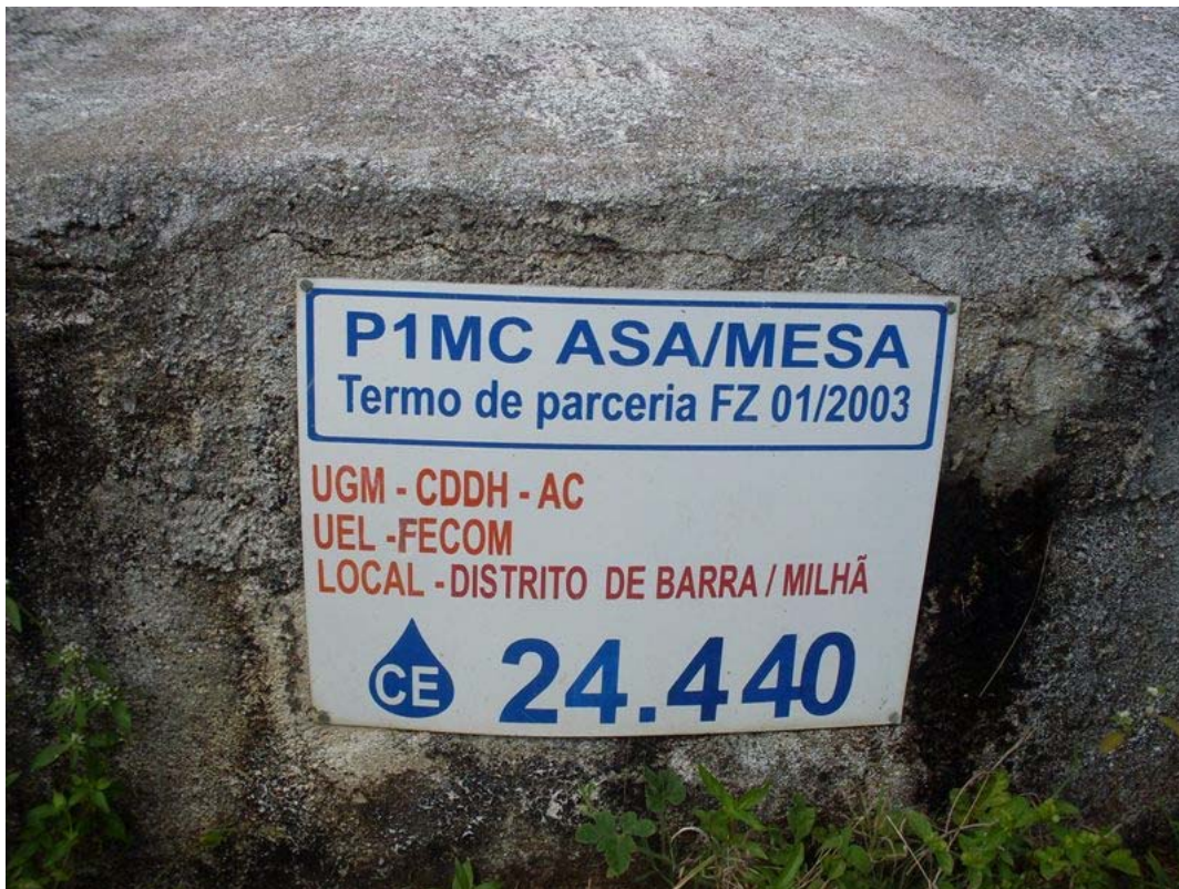
Fig. 4.158: Rainwater cistern in Barra 01.
