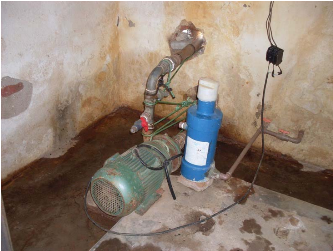
Figure 4.4: ETA Pumps for the elevated reservoir. Power = 7.5 HP.
