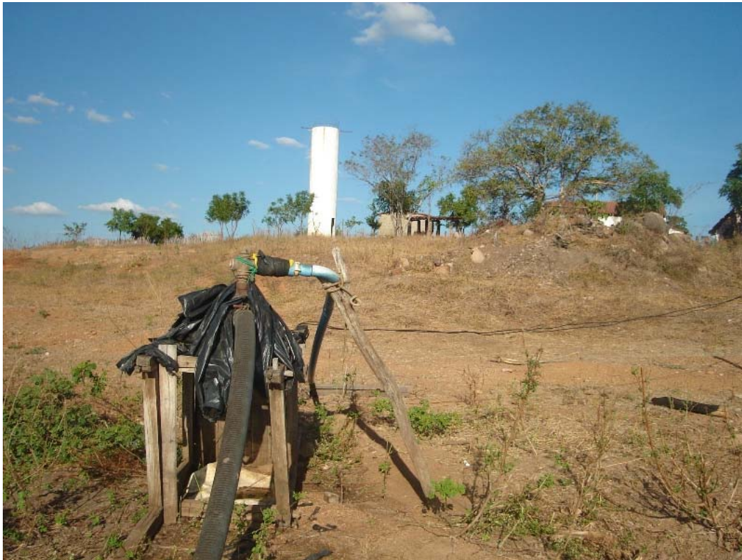
Figure 5.5: Water pumping at the João Vieira reservoir; an elevated reservoir in the back, which provides water to the community of Esperança.
