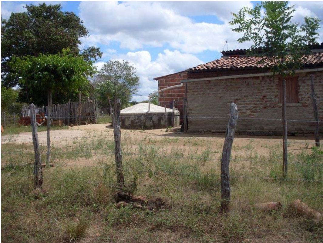
Figure 5.32: Rainwater cistern in the community of Deus me Ajude.
