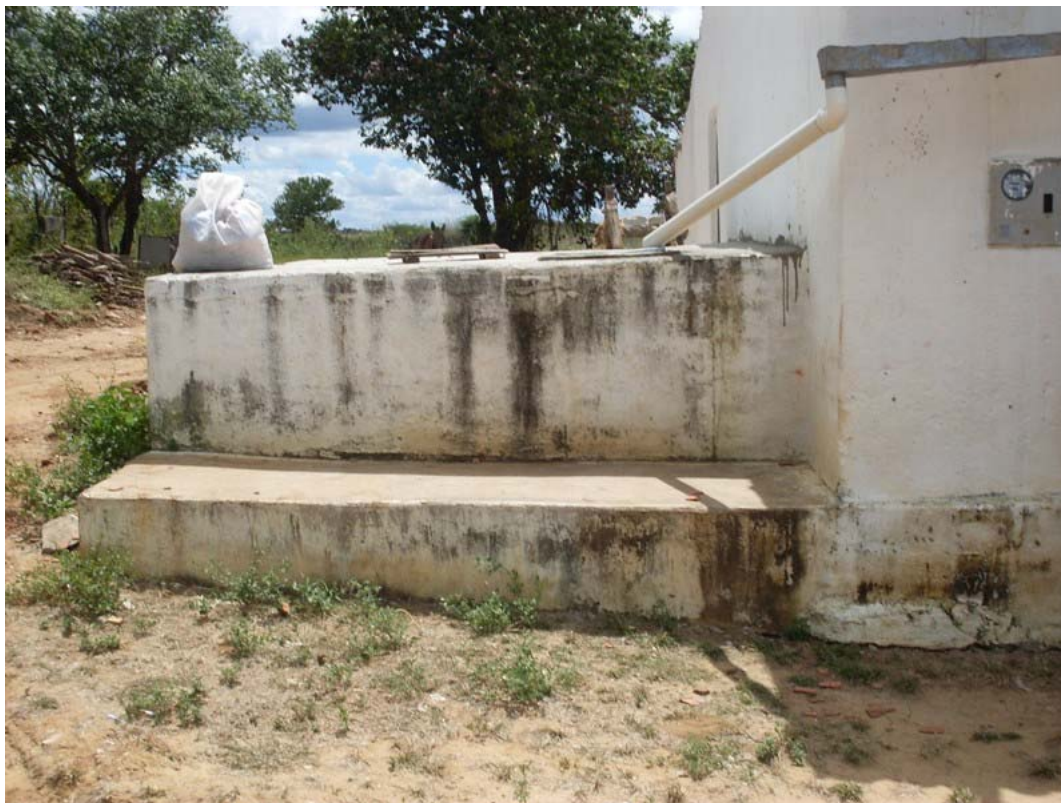
Figure 4.47: Private cistern at a home in Bom Alívio.
