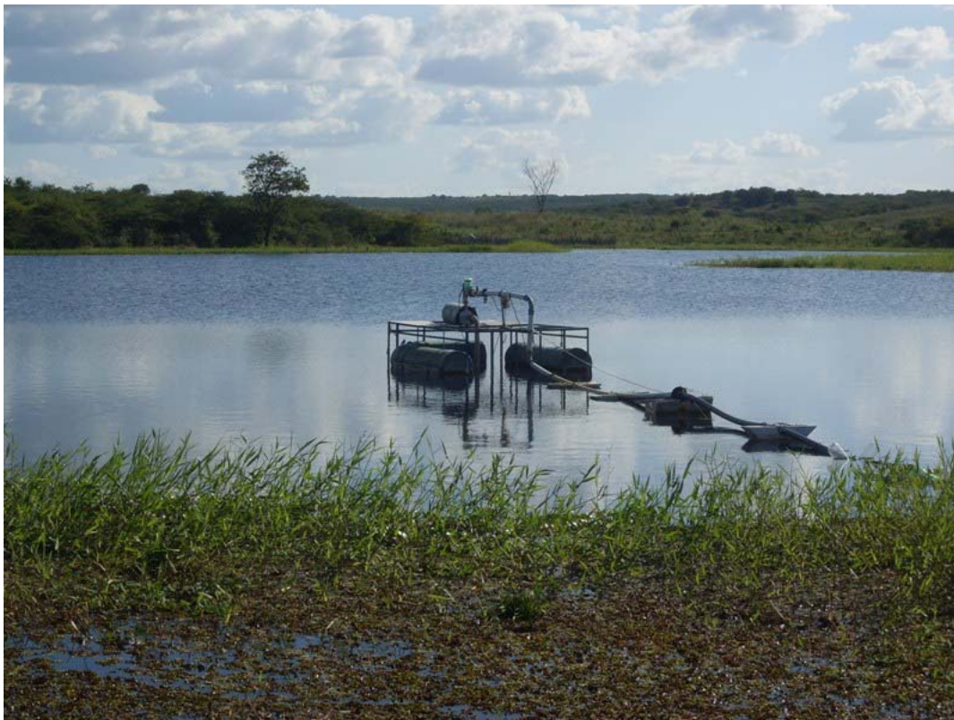
Figure 4.49: Floating water collection in the São Sebastião reservoir in Traíras.
