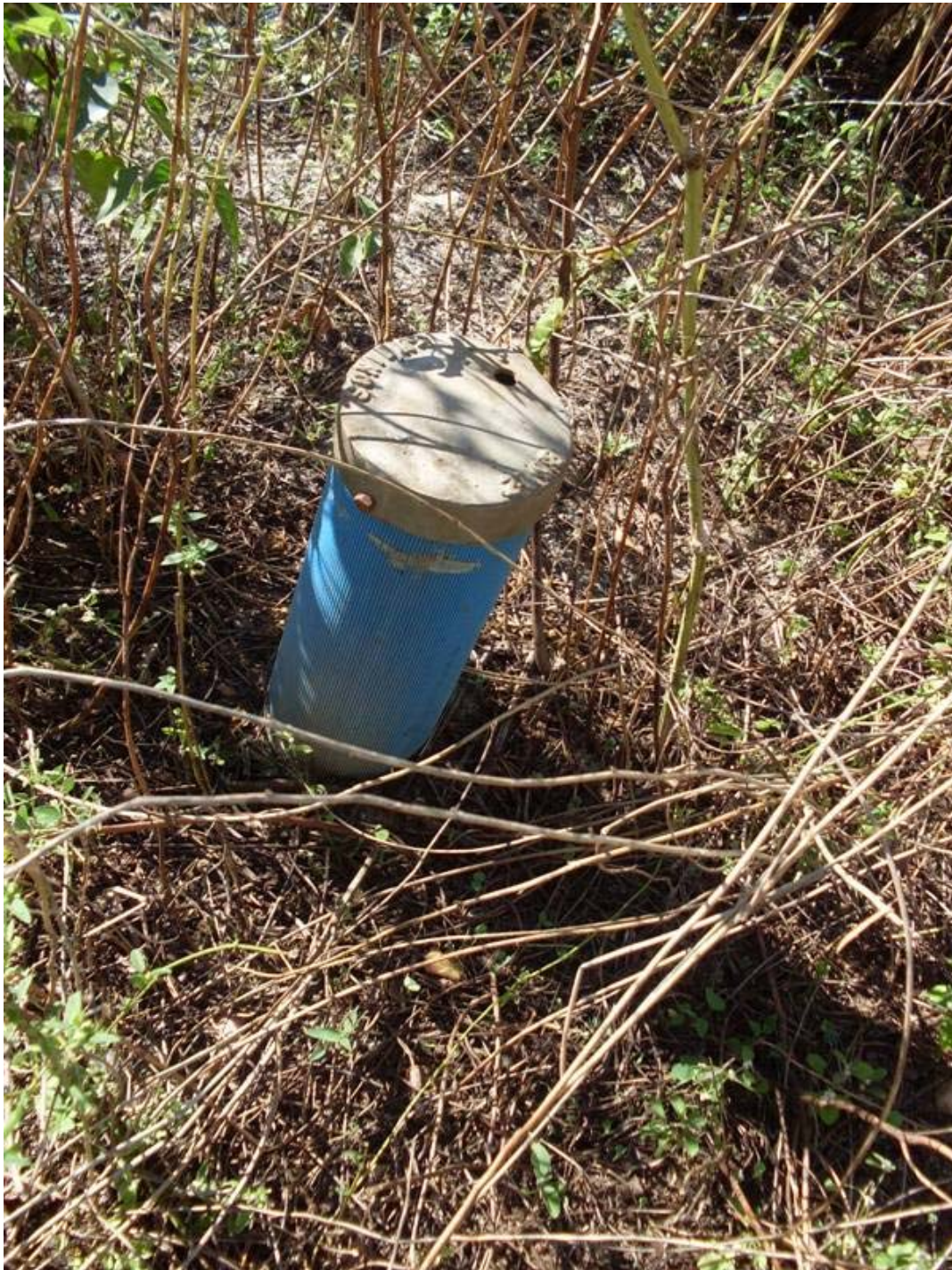
Figure 4.130: Deep well in Mr. Manoel Rodrigues Sila's property.
