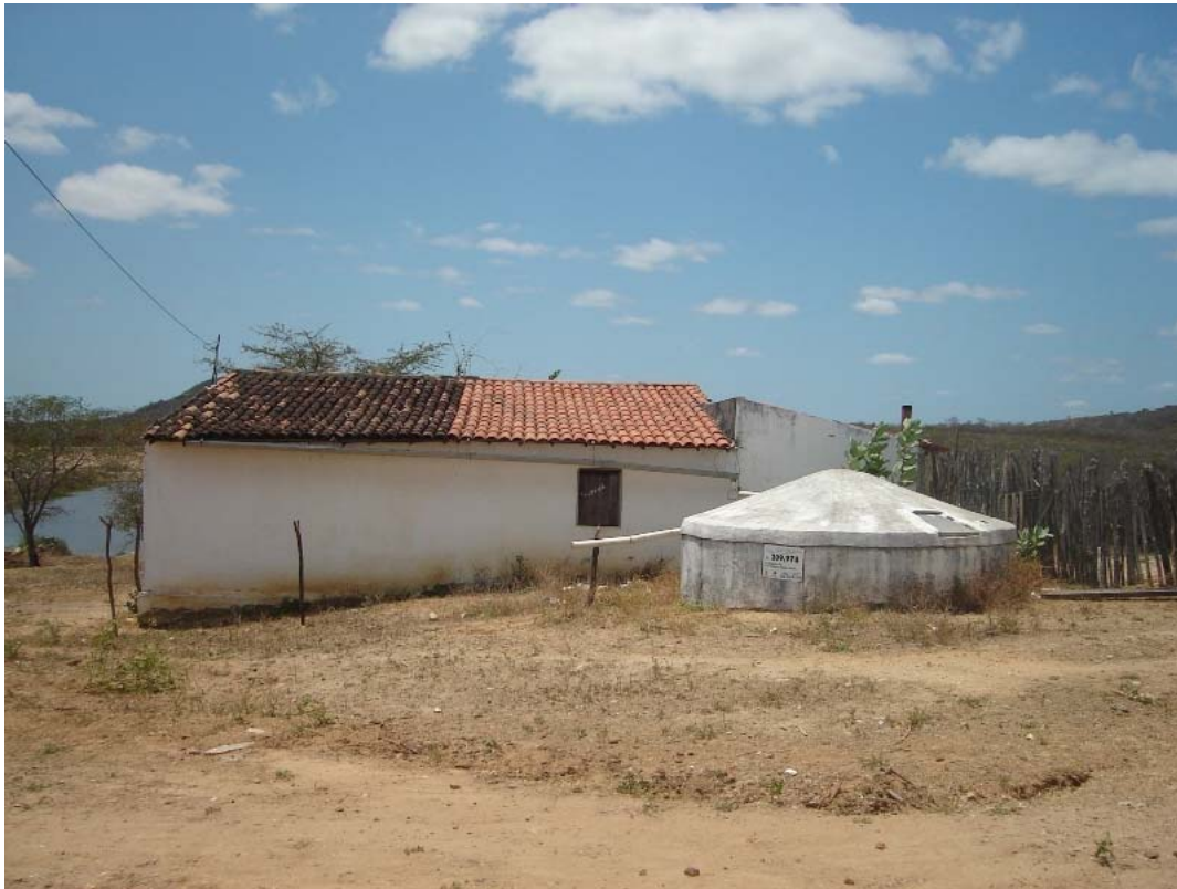
Figure 5.27: Rainwater cistern in Sítio Maré; it has leaked many times.
