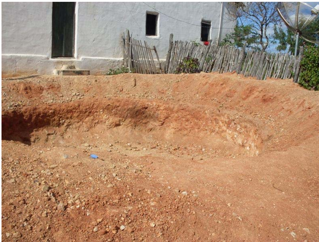
Figure 4.108: Excavation for the construction of rainwater cisterns (P1MC).
