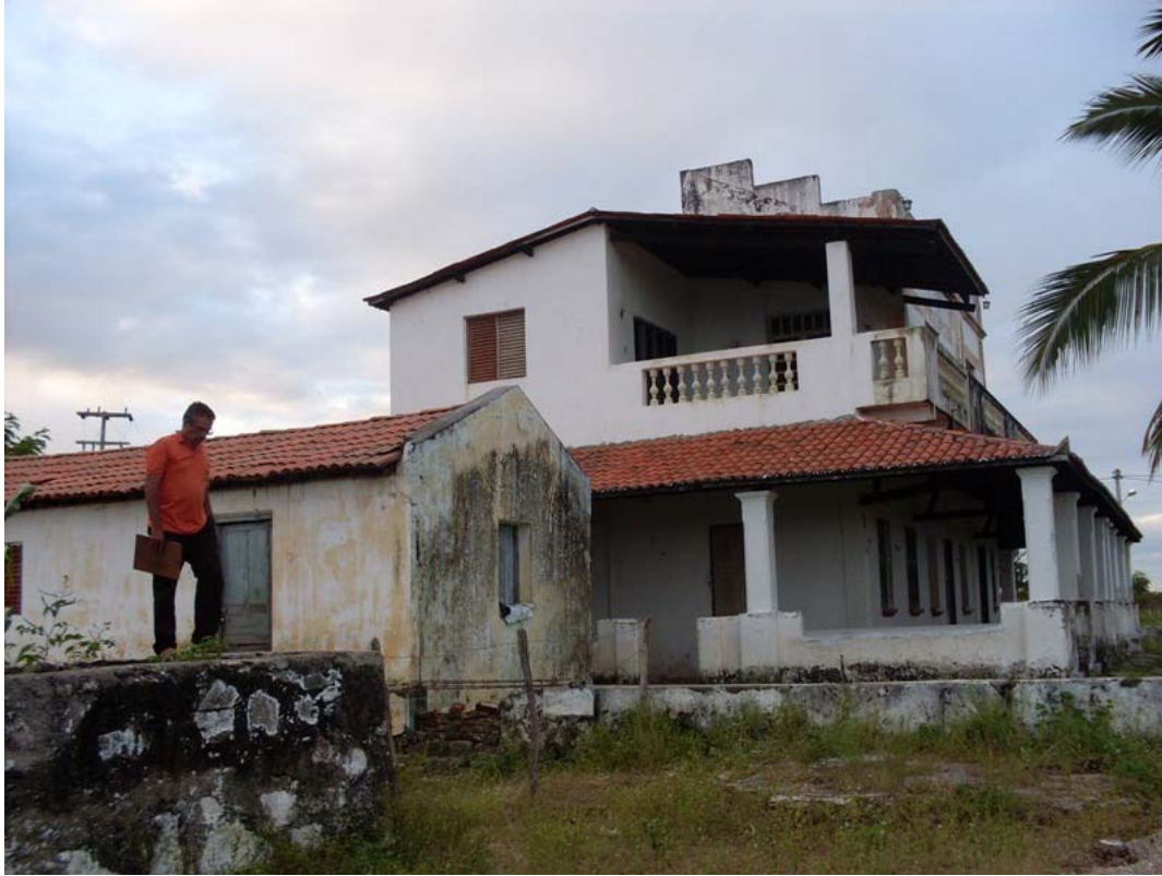
Figure 4.17: House in Grossos where the reservoir is located.
