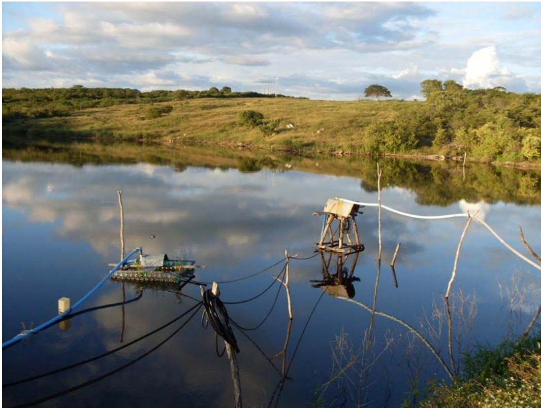
Figure 4.38: Water catchment from the Zezinho reservoir to homes in the community of Japão.
