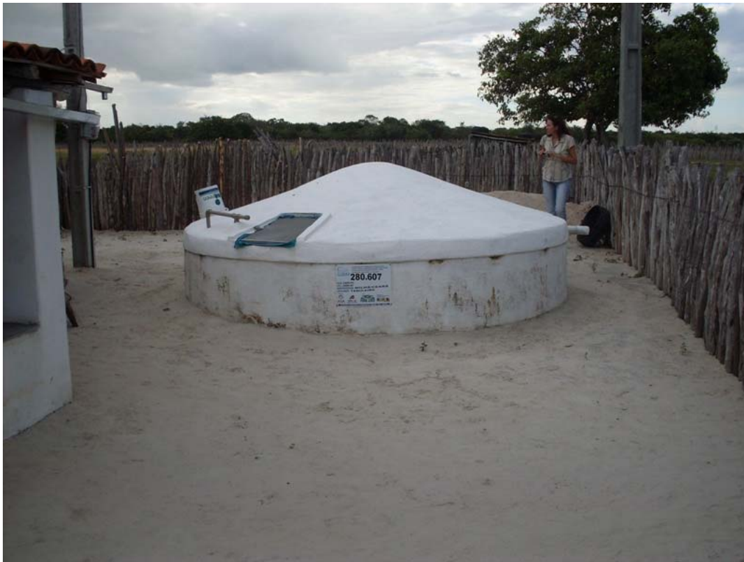
Figure 4.15: Rainwater Cistern at a home between Tabuleiro and Furnas.
