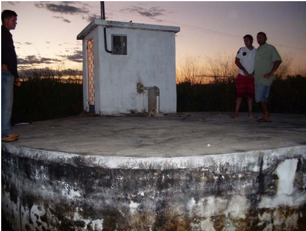
Fig. 4.155: An Amazon-type well and pump house that belong to the Barra system in Sítio Liberdade.
