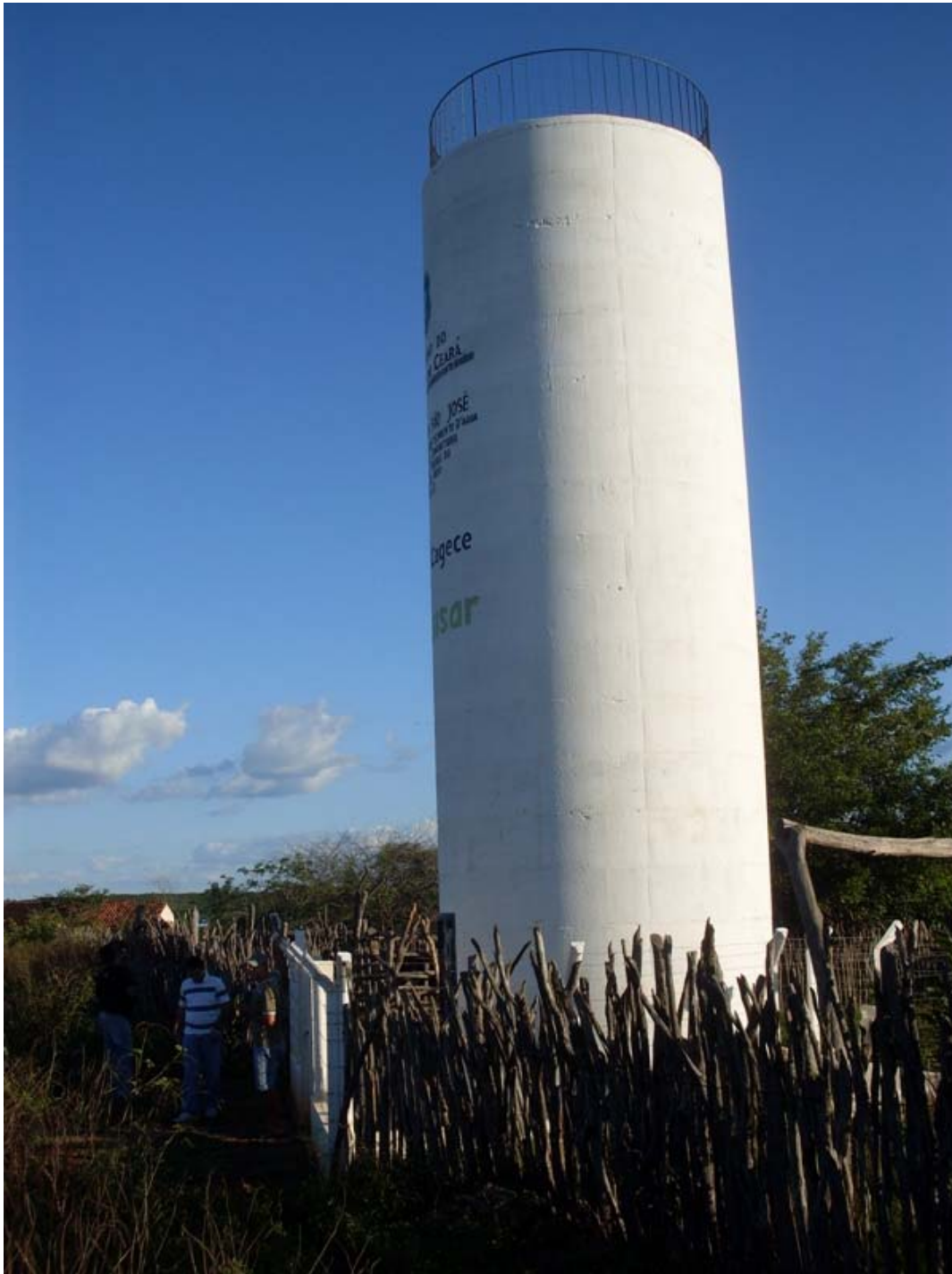
Figure 4.55: Elevated reservoir in Riacho do Meio.
