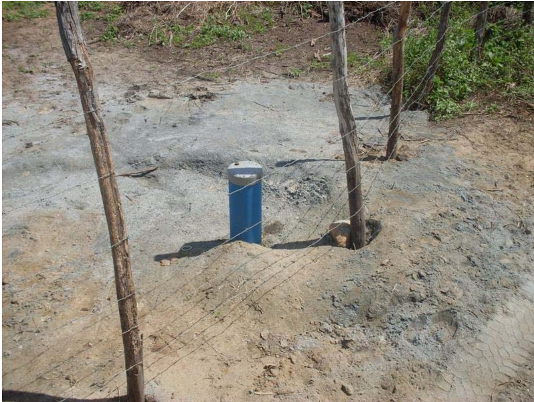
Figure 4.79: A deep well built in Esperança, flow rate = 3,000 L/h.
