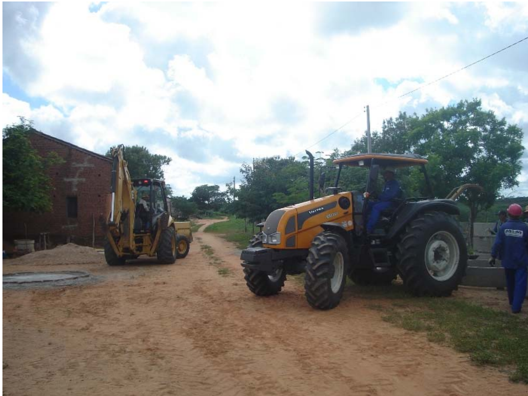
Figure 5.23: Operating machinery at Ingá's water supply construction site.
