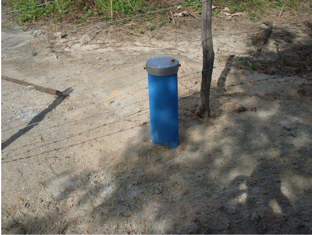
Figure 5.7: Deep Well in Bom Princípio. Flow rate: 3.3 m 3 /h.
