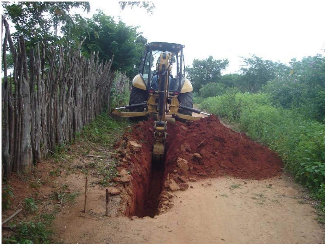
Figure 5.24: Scraper truck digging a pipe ditch in Ingá.
