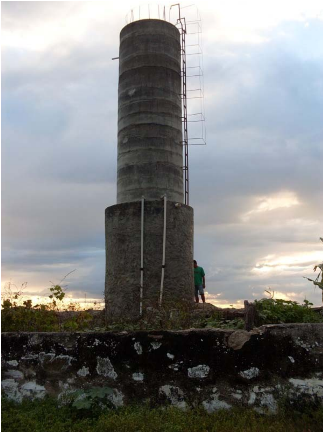
Figure 4.16: Grossos ground level/elevated reservoir.
