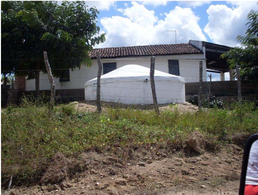
Fig.4. 148: Rainwater cistern in Almeixa
