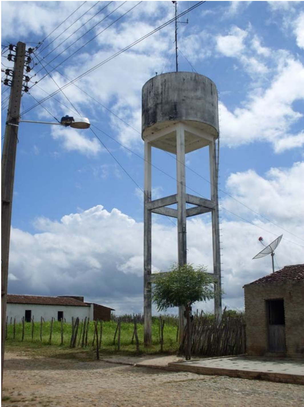
Figure 6.5: Elevated reservoir of the District of Carnaubinha. Vol= 55 m 3 .
