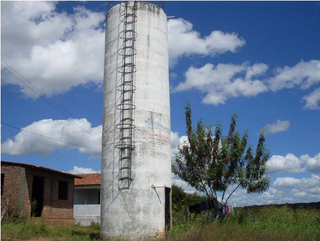
Fig. 4.183: Lagoa Nova's Elevated reservoir.
