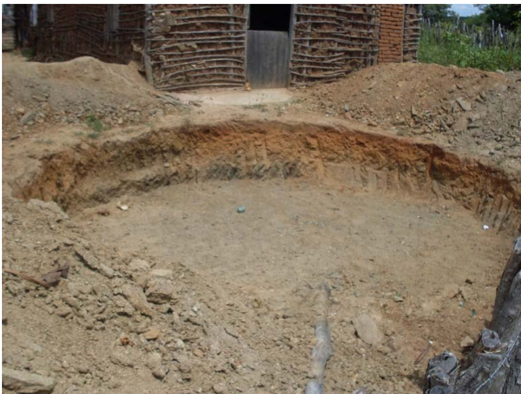
Figure 4.81: Rainwater Cistern under construction in Esperança.
