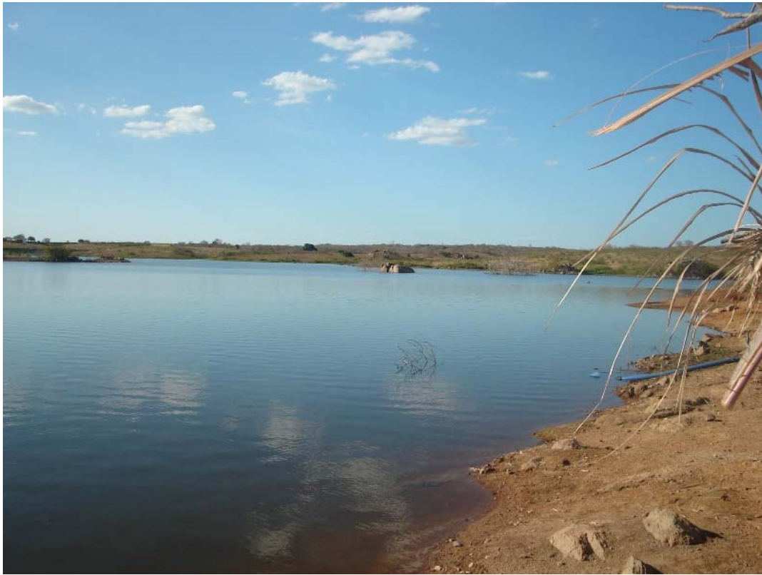
Figure 5.4: João Vieira Reservoir; on the far right, collection of water for Esperança.
