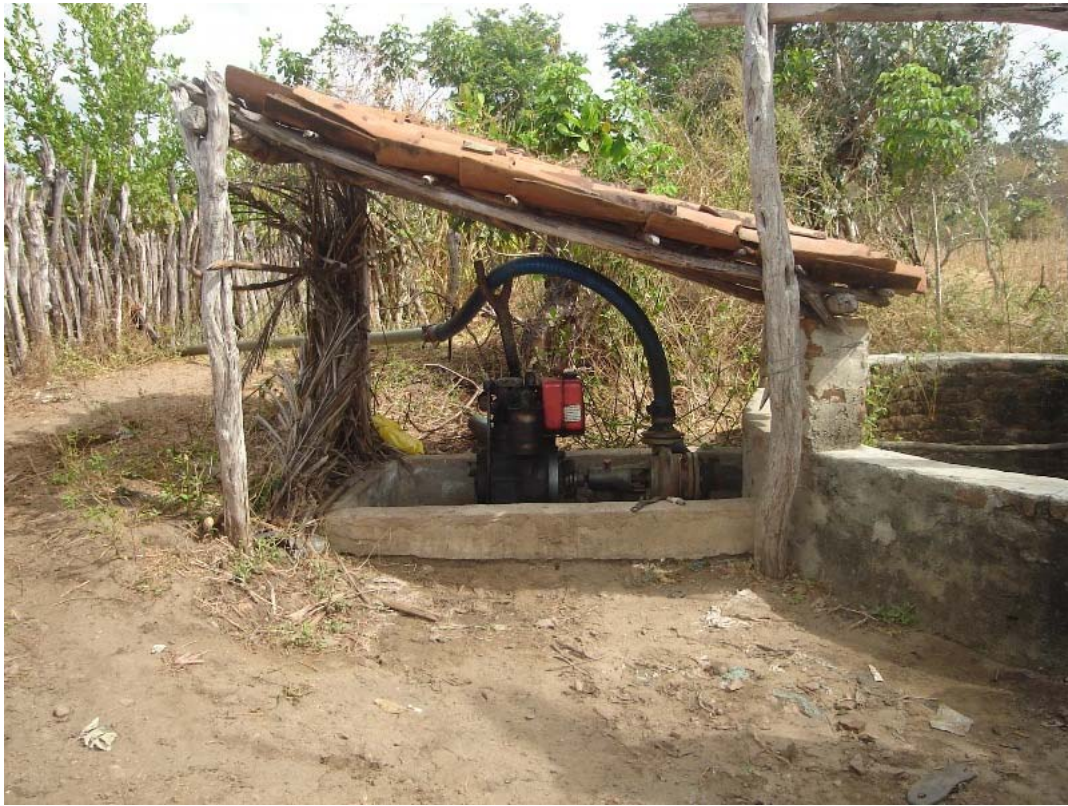
Figure 5.29: Diesel pump collecting water from the Amazon-type well for irrigation.
