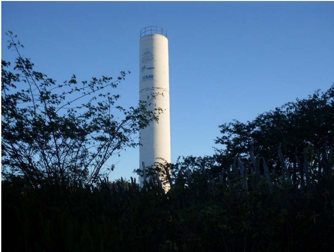
Fig.4. 150: Elevated reservoir in Barra 2.
