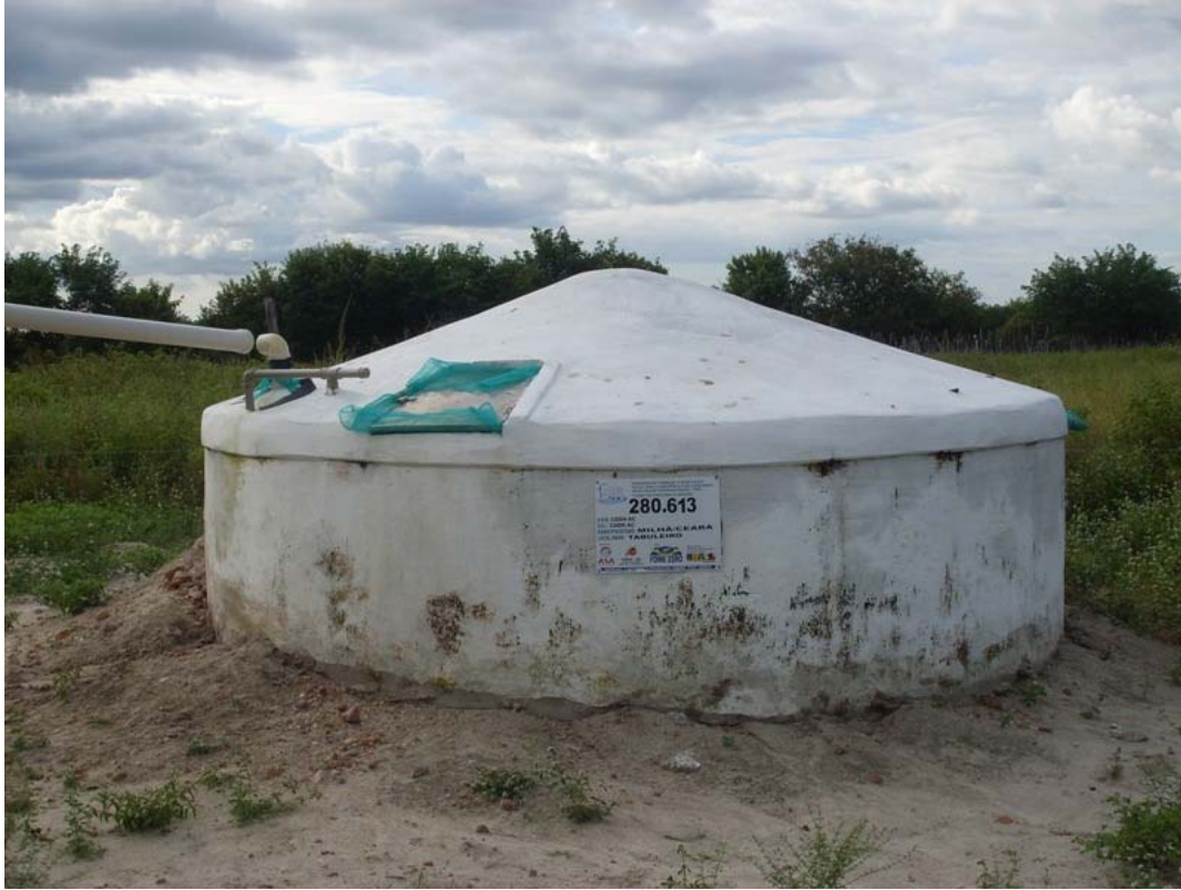
Figure 4.14: Rainwater Cistern in Tabuleiro.
