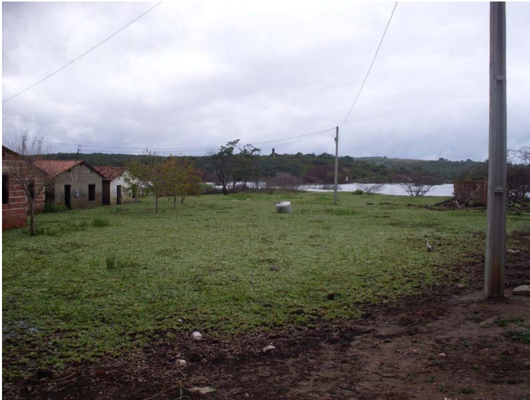
Figure 4.20: An abandoned filter on the banks of Antenor Pinheiro Reservoir.
