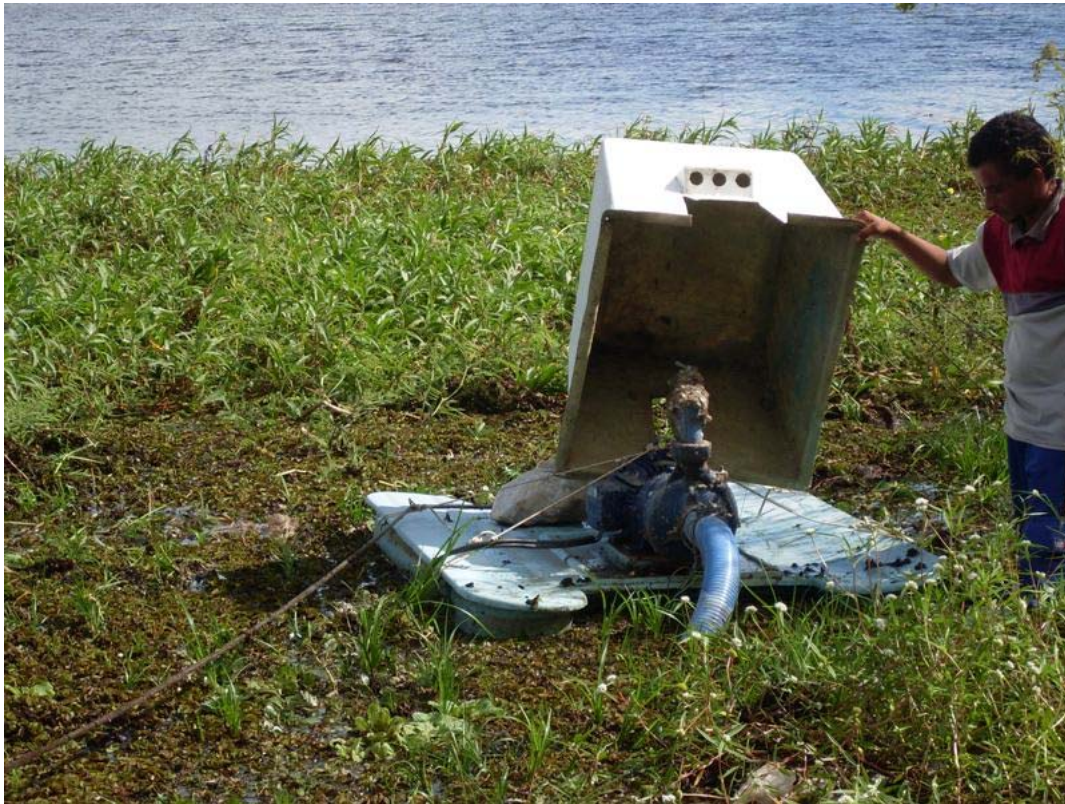
Figure 4.10: Catchment system used in the Berilópolis reservoir to supply Açude Novo, Alto Santo (Cabeça de Boi), Grossos, Furnas and Tabuleiro.
