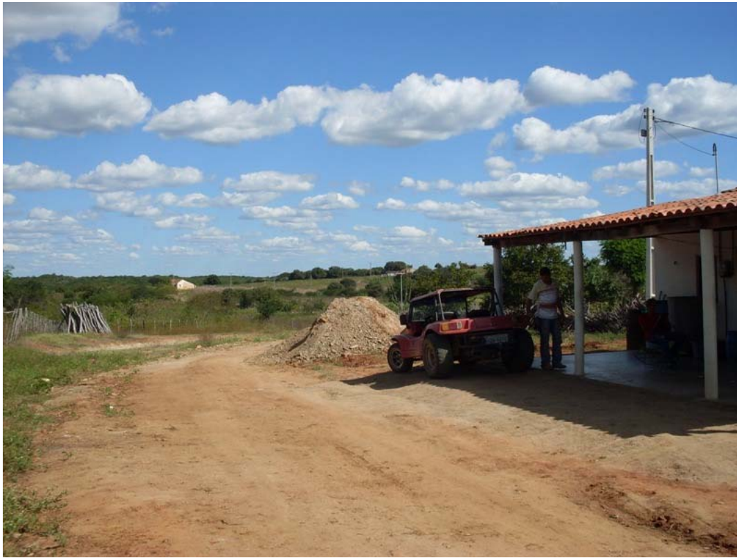
Figure 4.89: Rainwater Cistern under construction.
