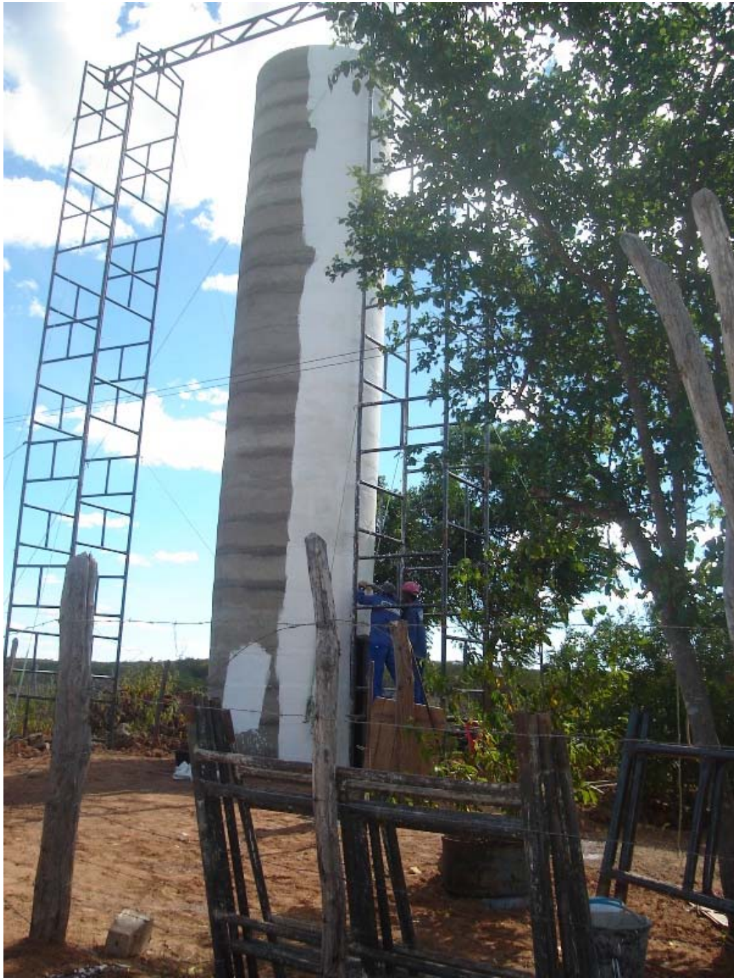
Figure 5.21: Ingá's Elevated Reservoir at the painting stage.
