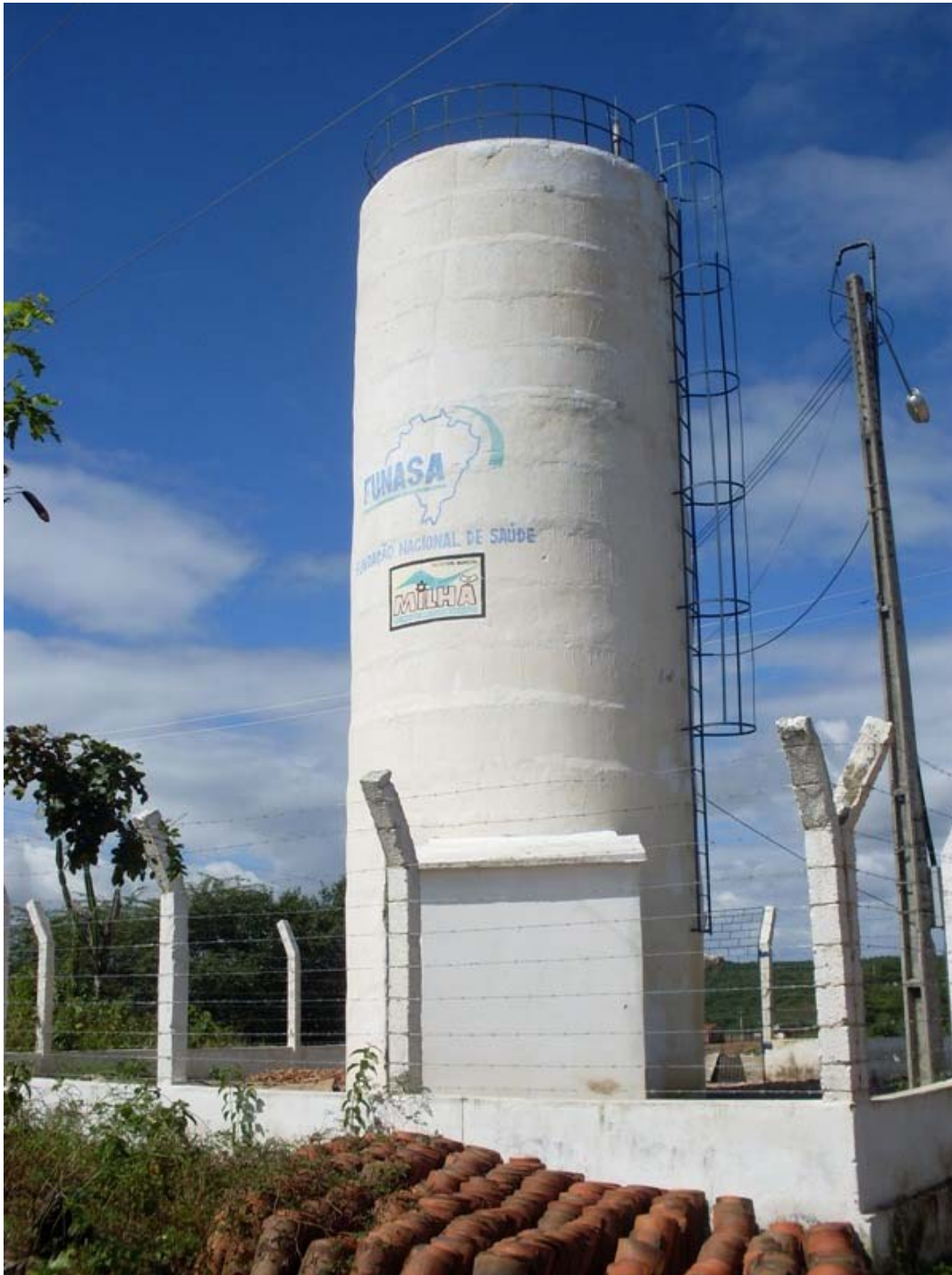
Figure 4.12: The Açude Novo Elevated reservoir which supplies Alto Santo, Grossos, Açude Novo and Tabuleiro.
