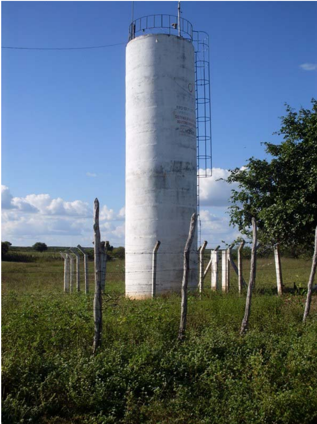
Figure 4.50: Trairas' Elevated Reservoir.
