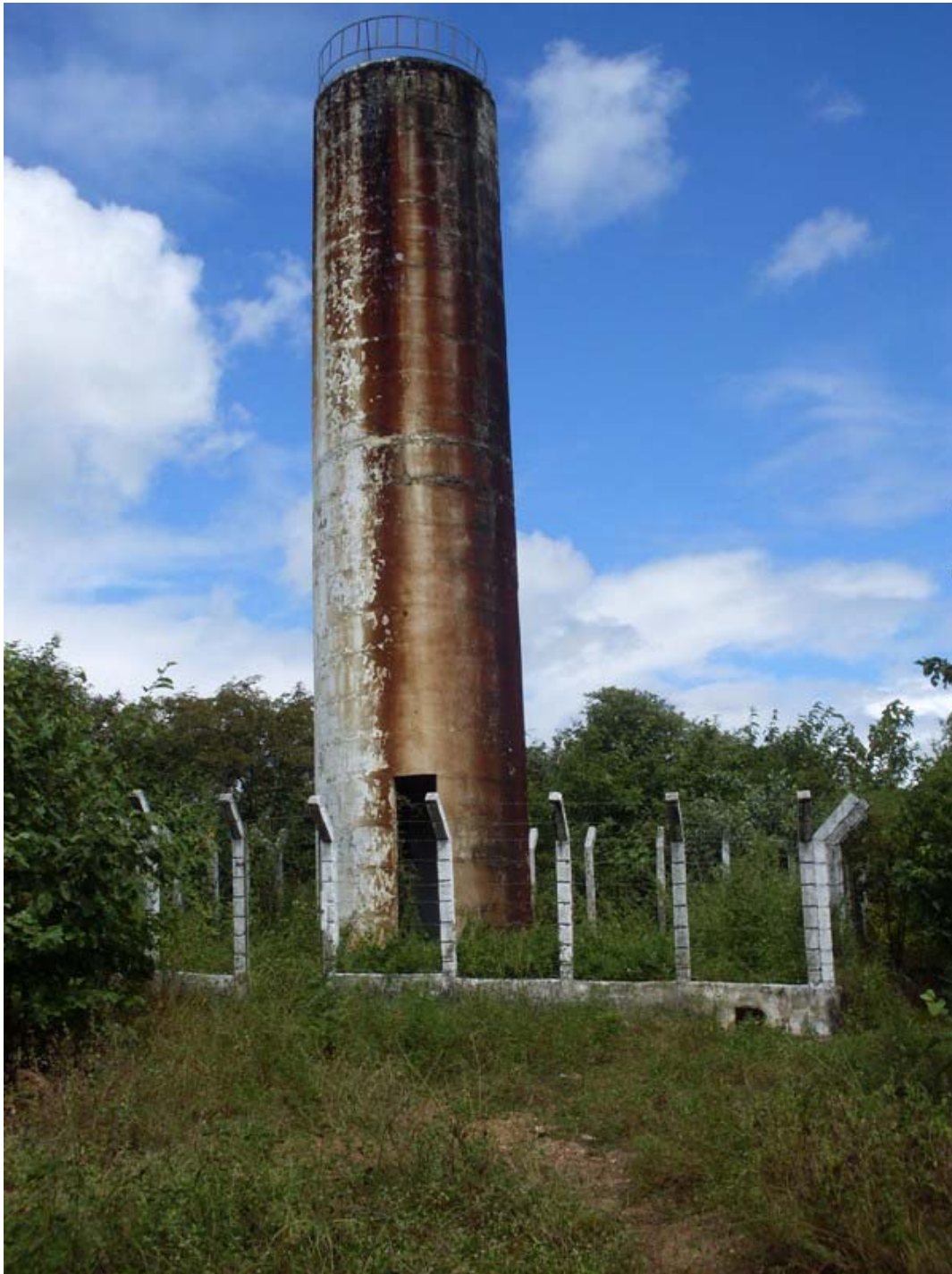
Figure 4.22: Elevated reservoir of the District of Ipueiras, currently isolated by the Antenor Pinheiro reservoir.
