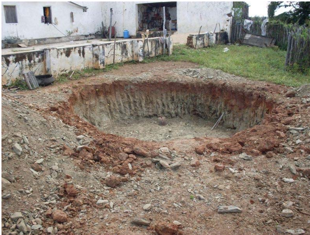
Figure 4.85: Rainwater Cistern under construction in Sabonete (P1MC).
