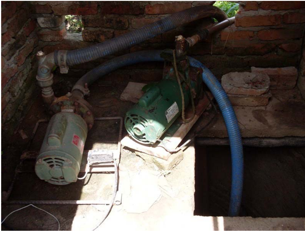
Figure 4.26: Pumps in Quandu's Amazon-type well, with different administrators and water charges.
