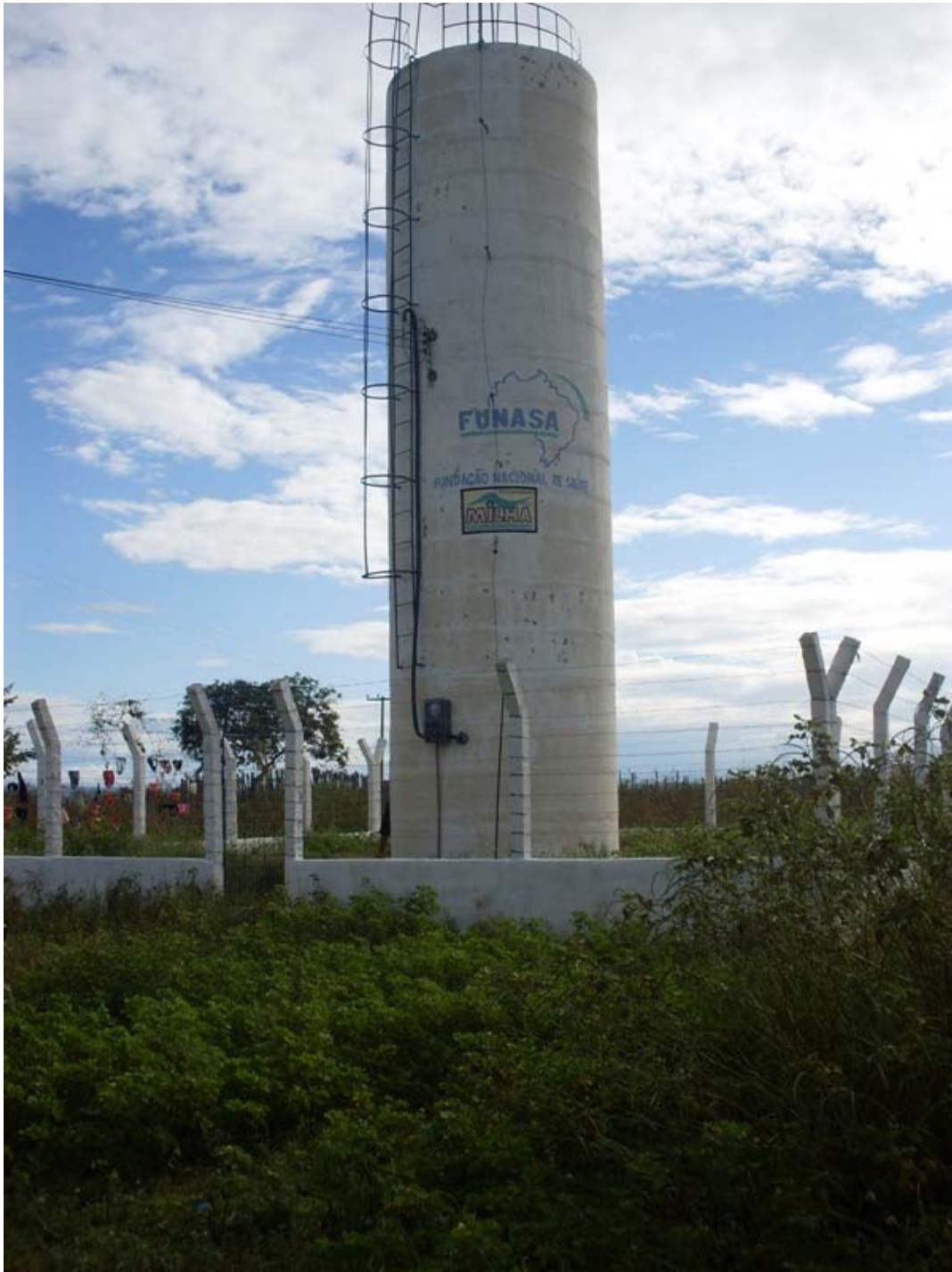
Figure 4.13: Tabuleiro's 21 m 3 elevated reservoir.
