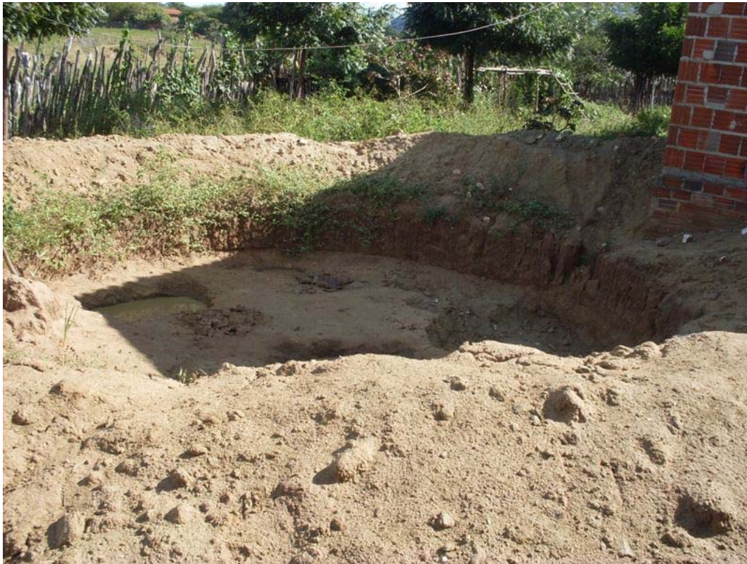
Figure 4.131: Excavations for the construction of cisterns under the 1 Million Cisterns Program.
