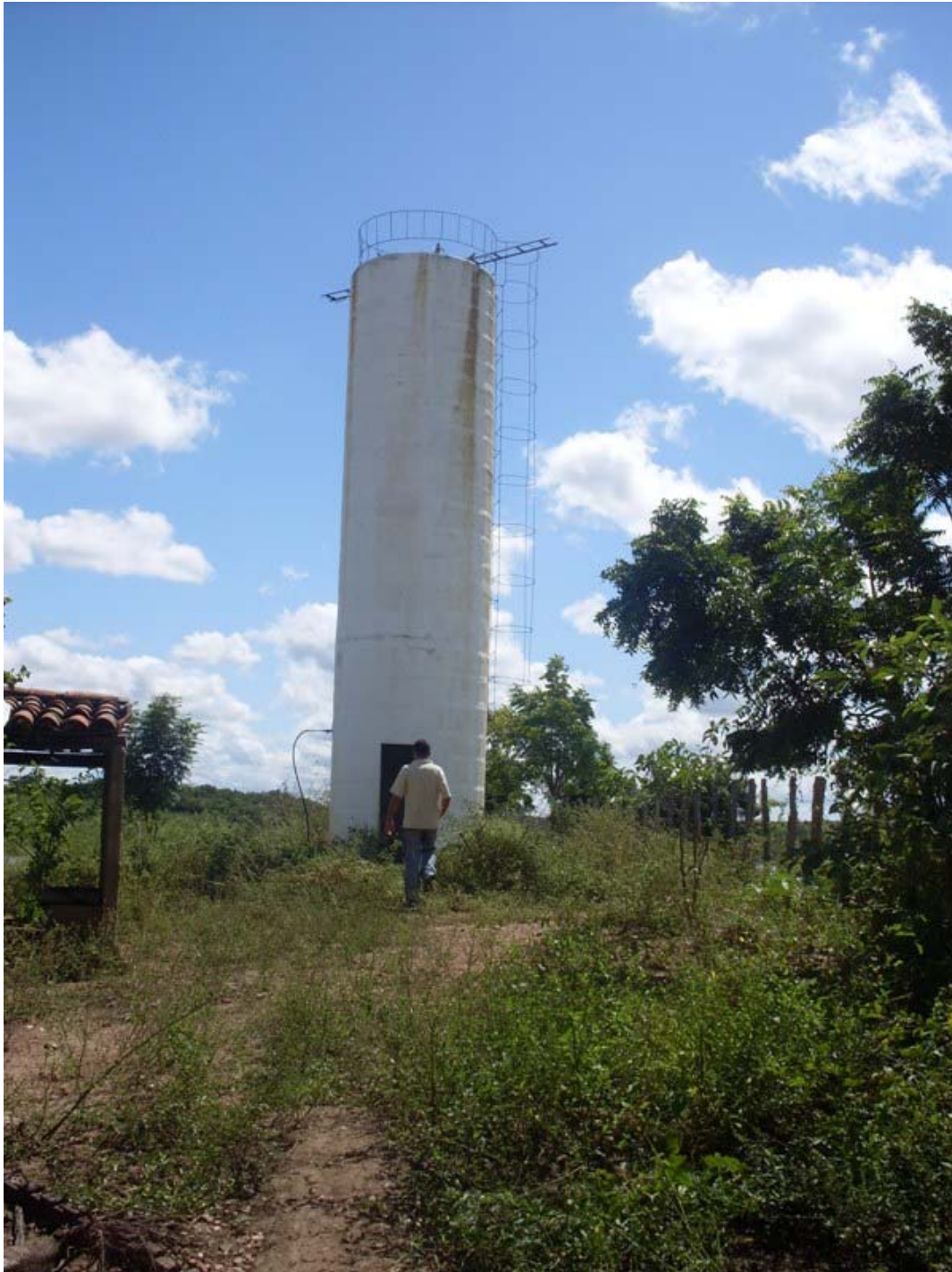
Figure 4.78: Elevated reservoir that provides water to ten homes in Esperança.
