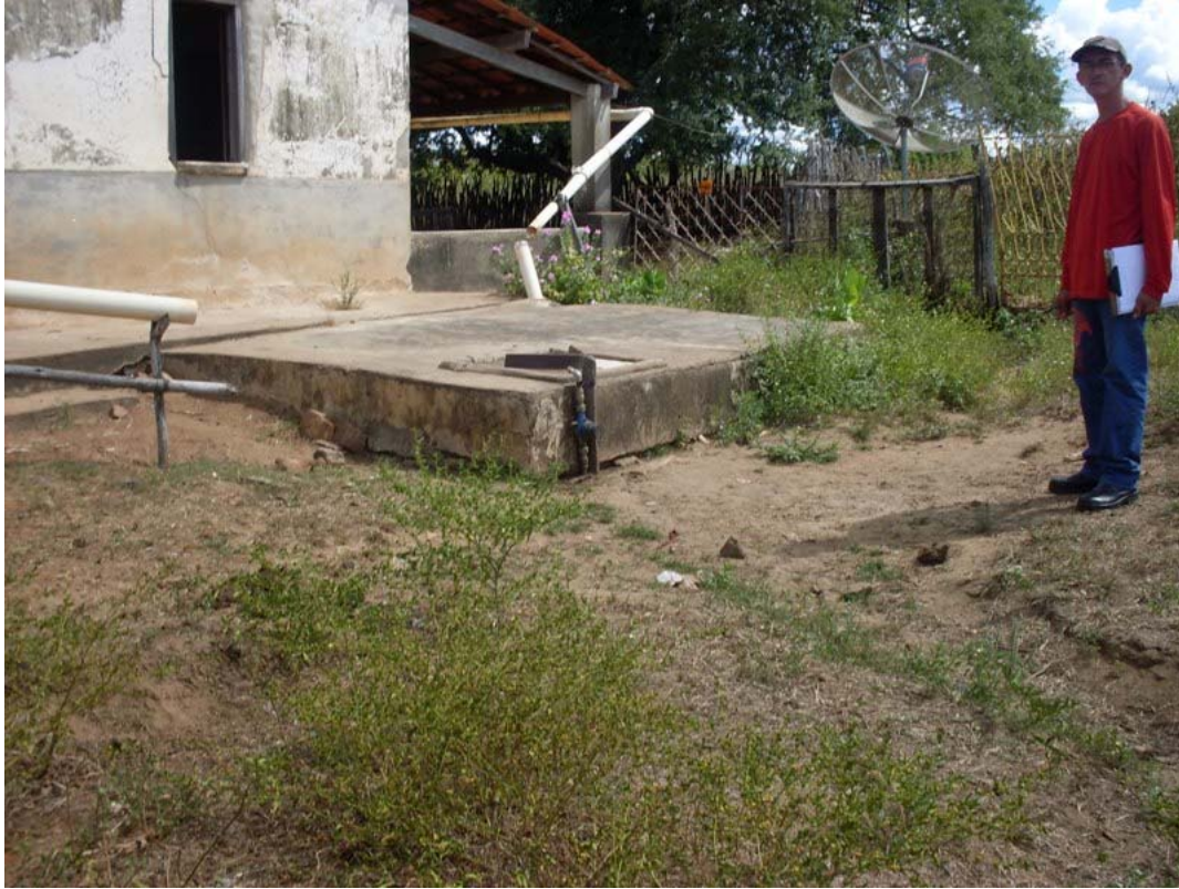
Figure 4.124: A prismatic cistern built in Sítio Açude by Milhã's Municipal Government.
