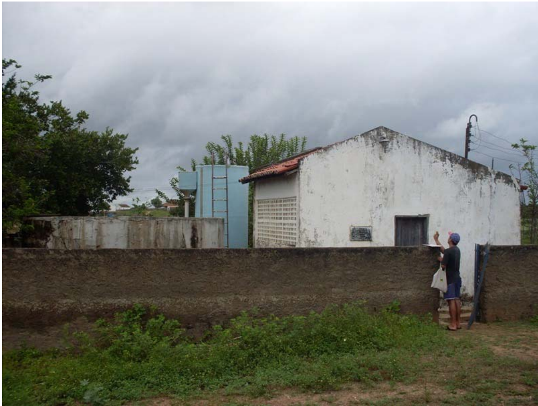
Figure 4.3: Carnaubinha's Water Treatment Station.
