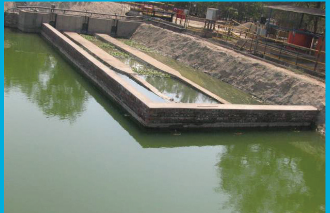
Use of wastewater for horticulture reduces the freshwater intake
